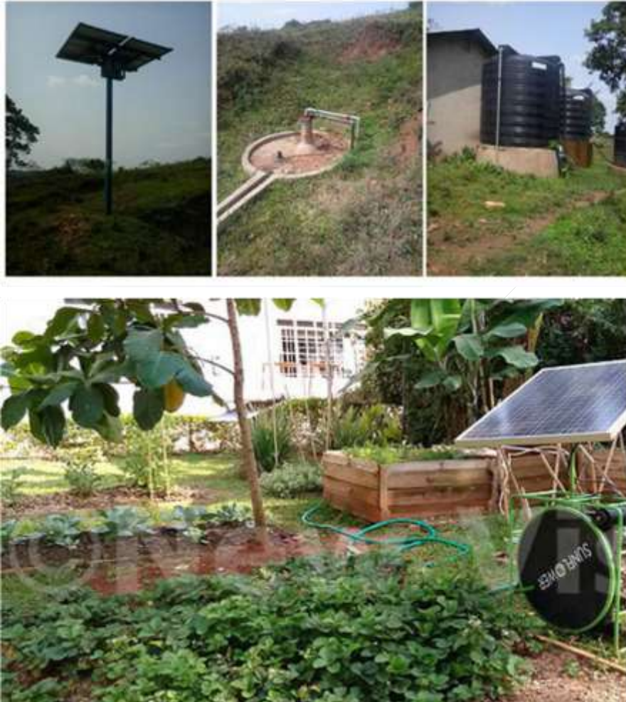
Figure 1 Solar powered irrigation: A solar powered abstraction adapted on a borehole (top); Future solar water pump distributed in Uganda by SolarNow Services (U) Limited (bottom)
