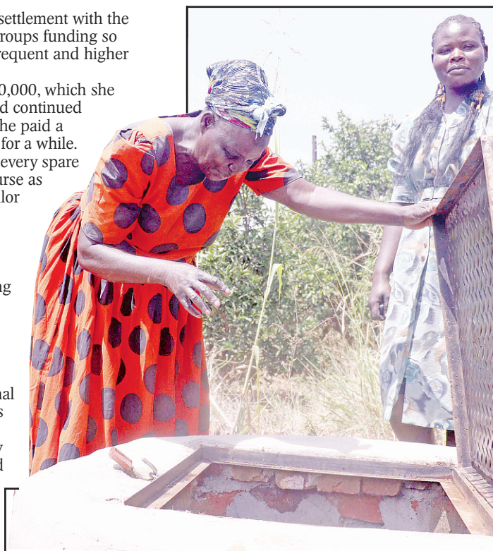
Izama used the VisionFund loan funds to dig a well that provides her water for irrigating her crops
