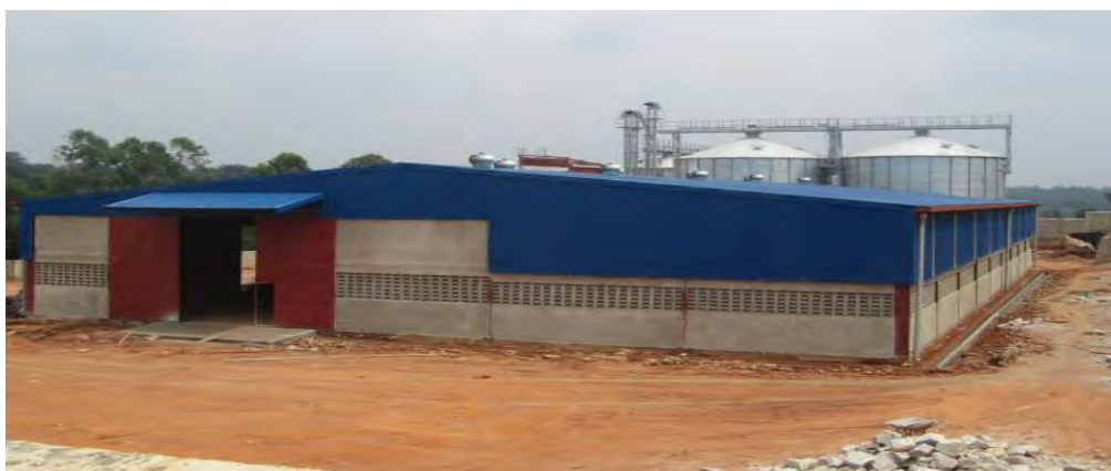
This Cereal processing facility in Mubende constructed with aBi support (Source: aBi VCD)
