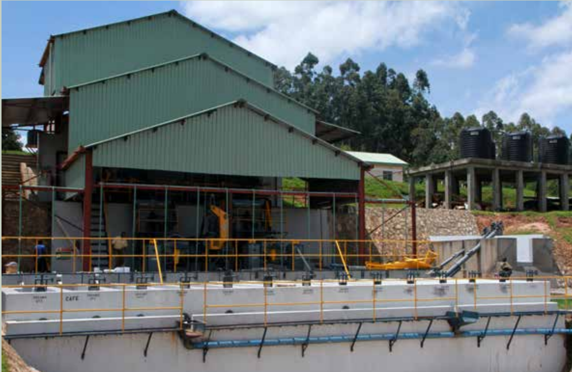
Kawacom's new White Nile wet mill facility, constructed with aBi support in Zombo District in Uganda's Northern Region.
